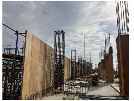
1F柱配筋•壁型枠建込
